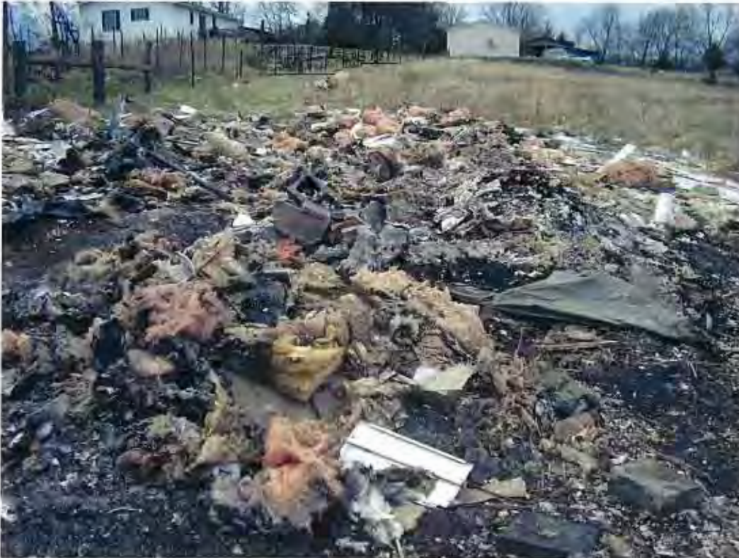
Date: 1/29/2008 Time: 12:54 P.M. Direction: north Photo by: S. Williams Exposure #: 007 Comments: charred demolition debris & ash
